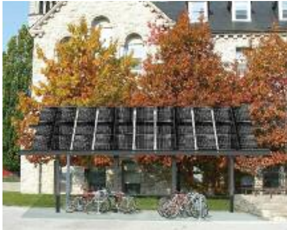
This manipulated image shows a solar-powered bicycle rack shelter, which was designed by fourth-year Mechanical Engineering students at Queen's. The 2.5-kilowatt apparatus would provide solar electricity for at least 30 years, while sheltering parked bicycles and generating a respectable return on the capital investment.
